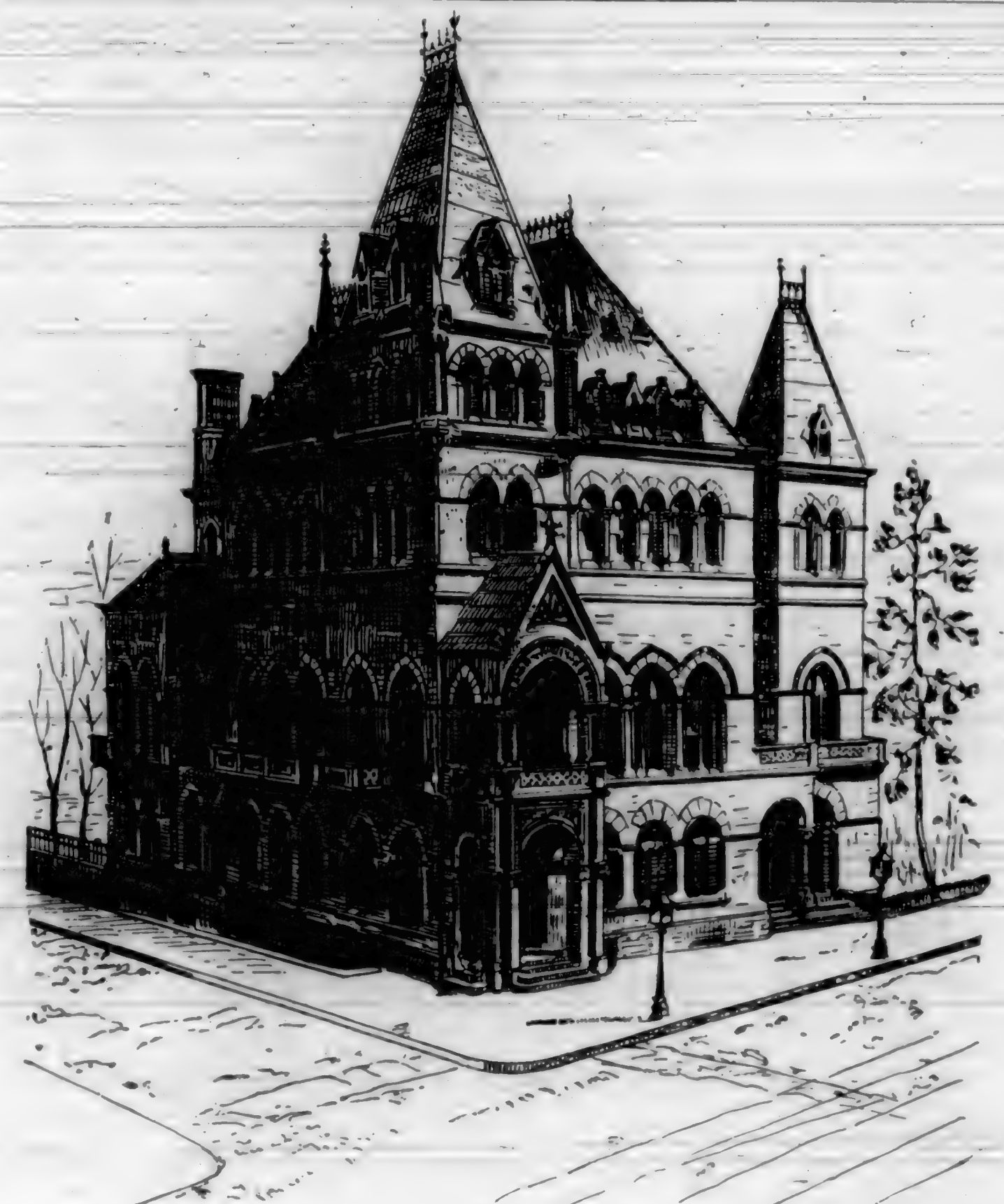
PLATE I.—DRY DOCK SAVINGS BANK.
