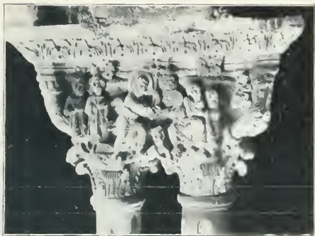
CAPITAL FROM THE CLOISTER, MONREALE
