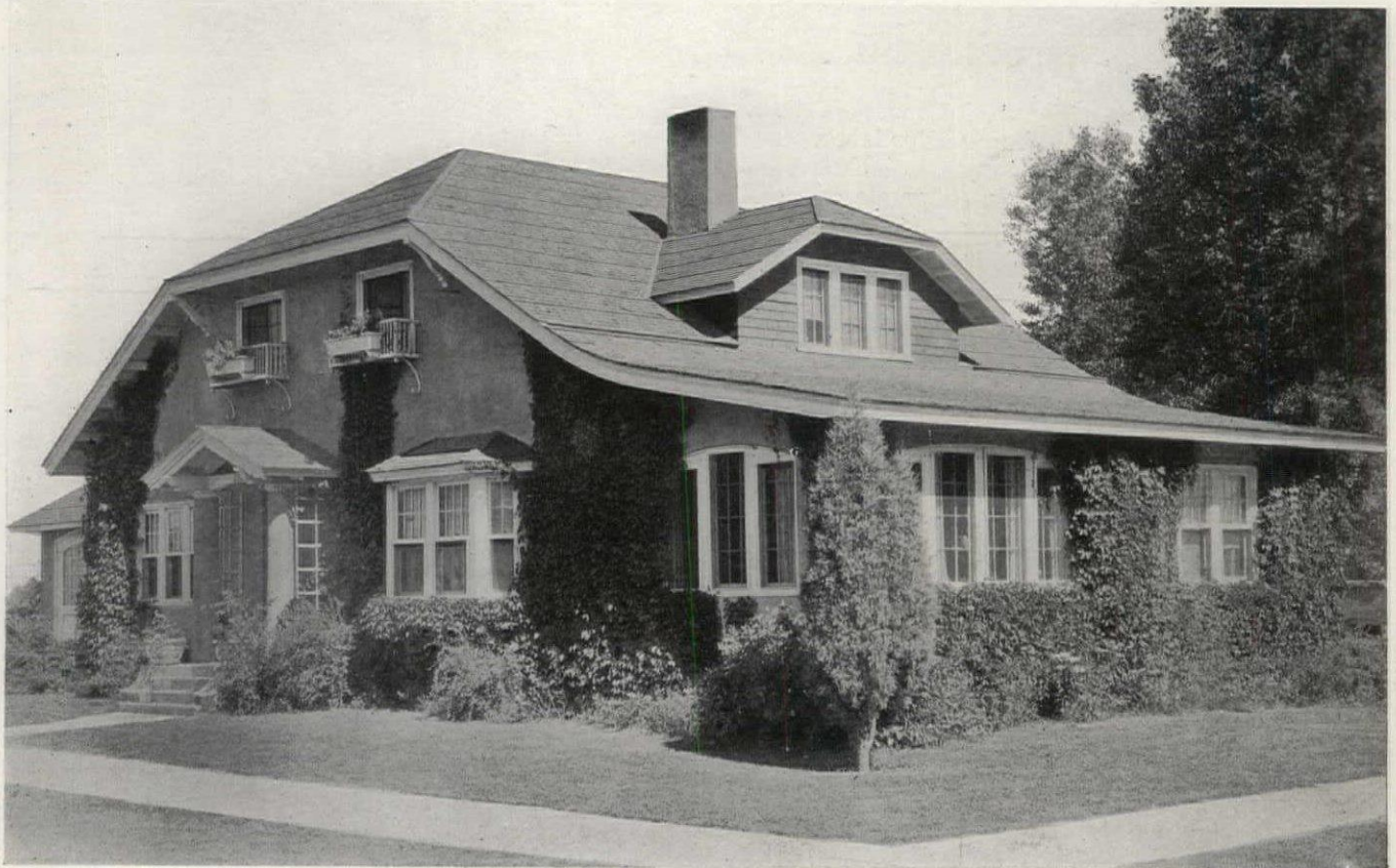
Note attractive sun porch in the Carlile house below, and interesting roof surface secured by doubling every sixth shingle course
