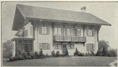
Res.—Mrs. Wm. B. Green, 133 Steele Road, W. Hartford Conn. Architect—Russell F. Barker, 43 Ann St., Hartford, Conn. Gen'l Cont.—W. A. Wilcox, 327 Trumbull St., Hartford, Conn. Stucco Contractor—Peter Leone Bishopric Stucco Base used on Exterior
