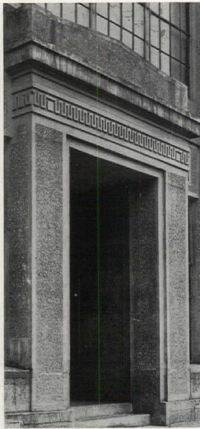
Fig. 2. Detail of entrance showing good effect of bush hammering, (the rougher surface) in contrast with smooth bands made by carborundum rubbing and filling of gray cement mixture. Fig. 3 below
