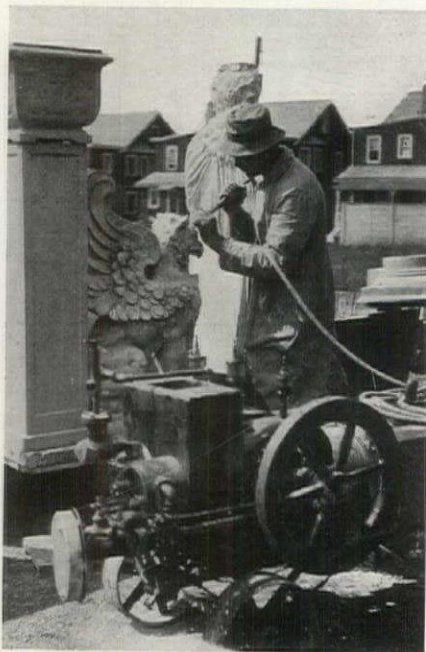
Cast ornamental concrete is given a variety of surface finishes by use of pneumatic tooling machines. Below is a concrete barn with white cement wash surface
