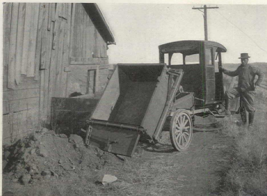
The Ford outfit showing the way tail gate operates with dirt load
