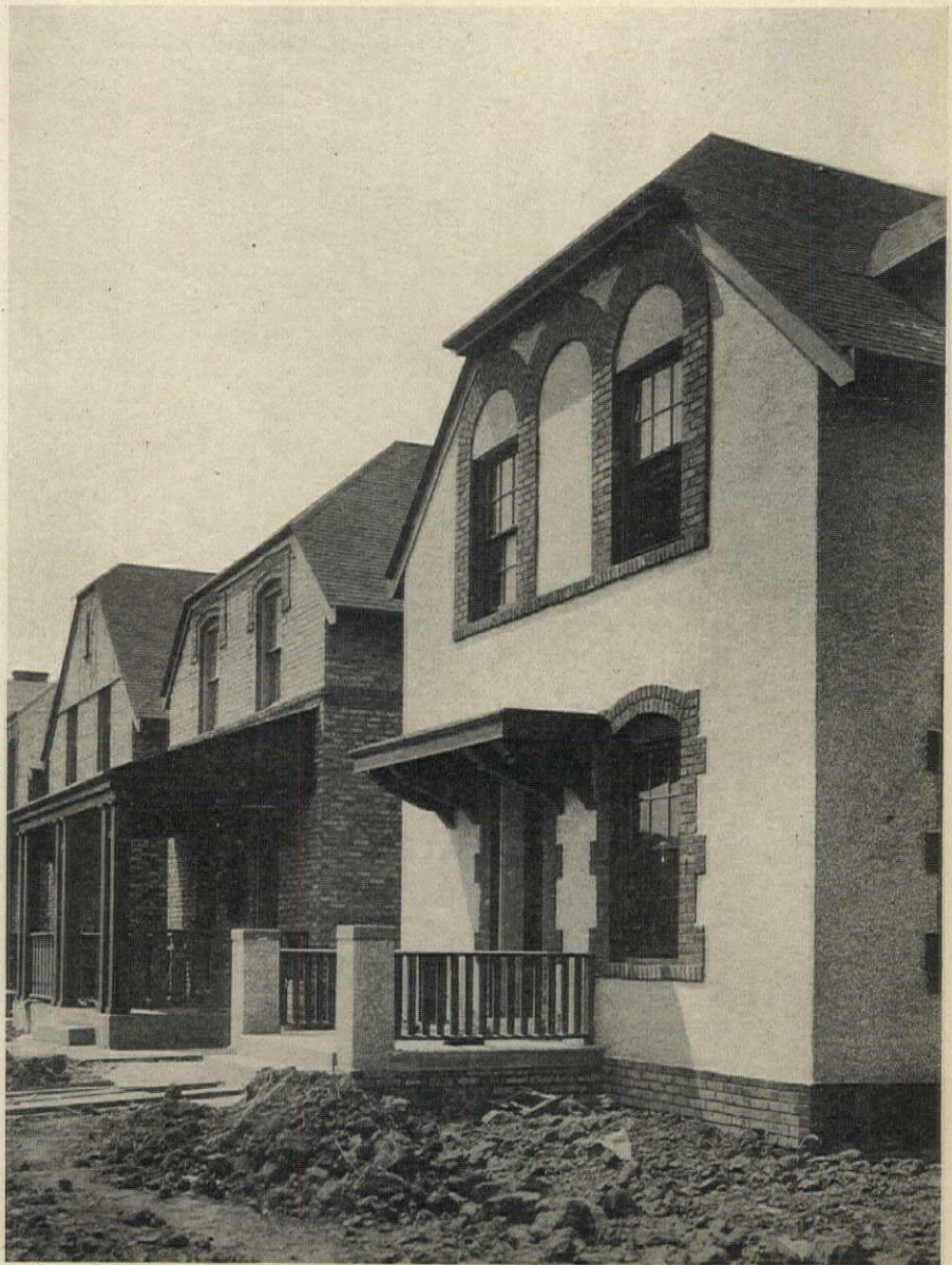
Stair balusters are 1 x 4 sawed boards
