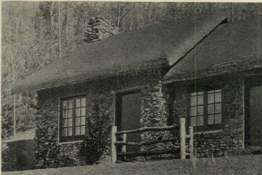
A thatched roof effect with mineral surfaced asphalt shingles. Note the texture given by the torn edges
