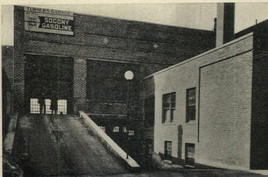
Garage on inside lot with narrow frontage to street with up and down ramps together. Note detail at left. George N. Meserve, architect
