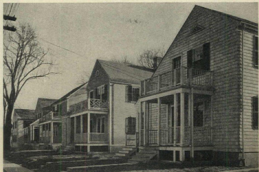
A second type of plan for 6 room single house. Note everything is contained in rectangle, insuring economy
