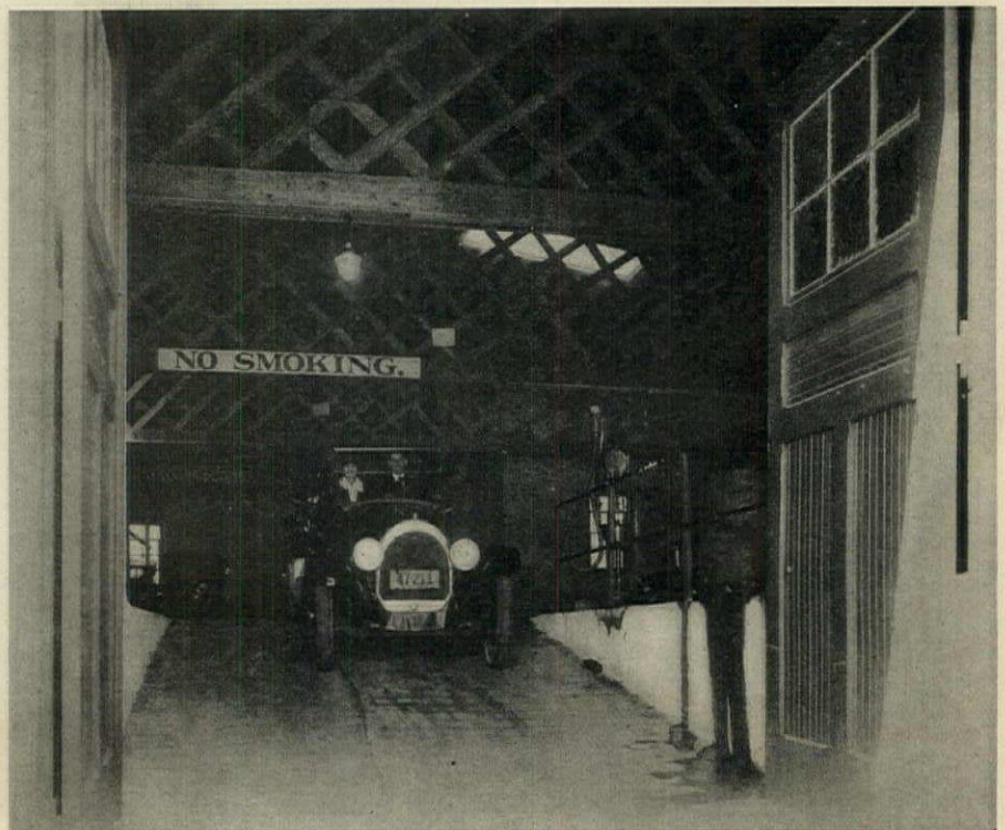
Ramp to upper floor of garage with ground level between floors. Note the lattice truss roof
