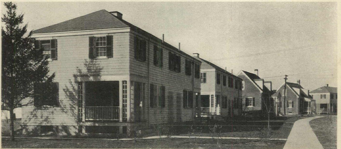
This Government housing development at Quincy, Mass., was built by Casper Ranger Construction Co. The houses were designed by James E. McLaughlin, architect; the town plan by Herbert J. Kellaway, landscape architect, and the engineering work by Ernest W. Branch, engineer. Walter P. Moulton, general superintendent
