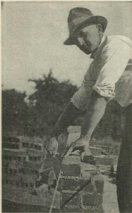
The pictures at right and left show operations in laying header and stretcher. Note that it is easier to lay a stretcher
