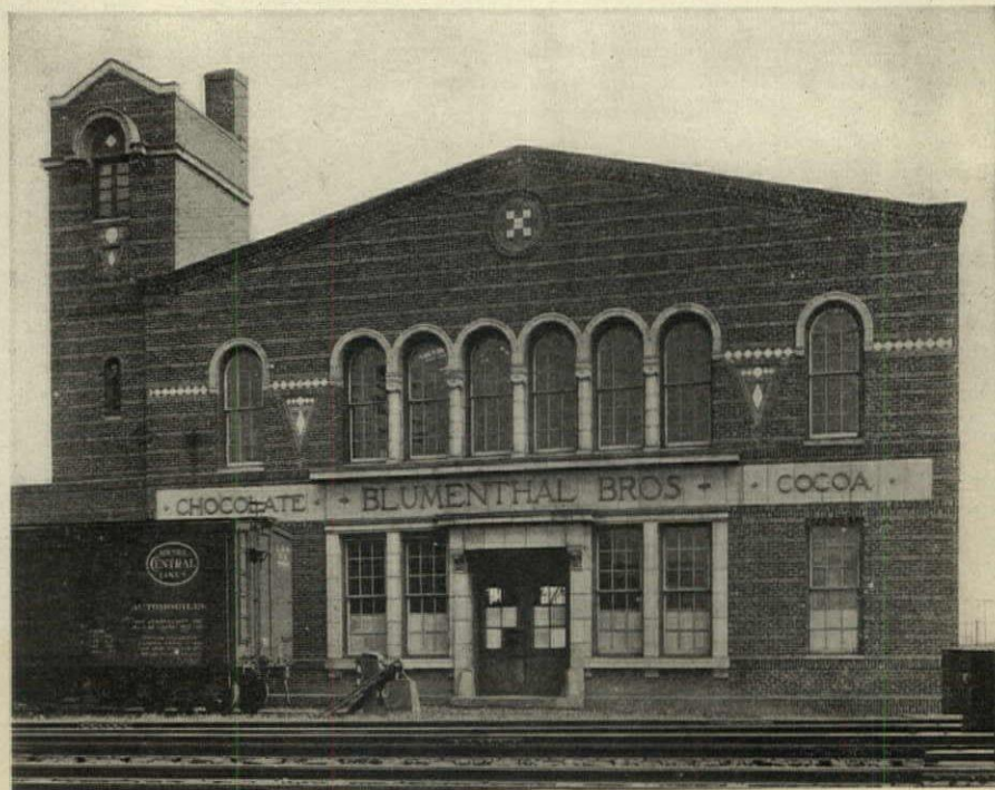
A factory near Philadelphia in which common bond has been used as decoration. The strong horizontal lines are header courses laid in different colored brick. Stearns & Castor, architects
