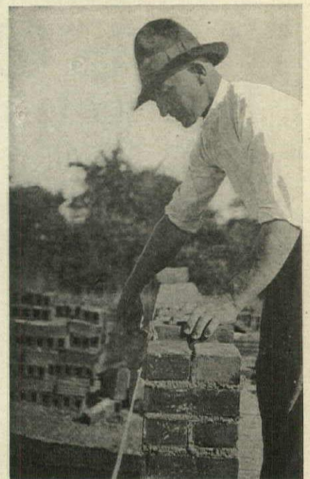
The pictures at right and left show operations in laying header and stretcher. Note that it is easier to lay a stretcher
