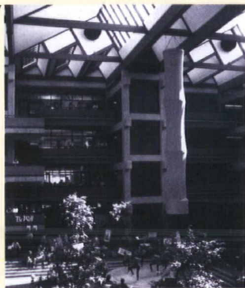
7 & 8. Hanging fabric tubes in the atrium of the Bateson Building were intended to counteract stratification of the air temperature. In practice, this turned out not to be an issue, and the casual observer is left wondering if they were meant to function more as legible signs of the designer's concerns vis-a-vis systems and 'energy flows'. The circulation walkway has in some places compromised the privacy of the office workers on the internal edge. Employees have constructed ill-placed partitions and window coverings, and as a result, the atrium daylight source has been blocked
