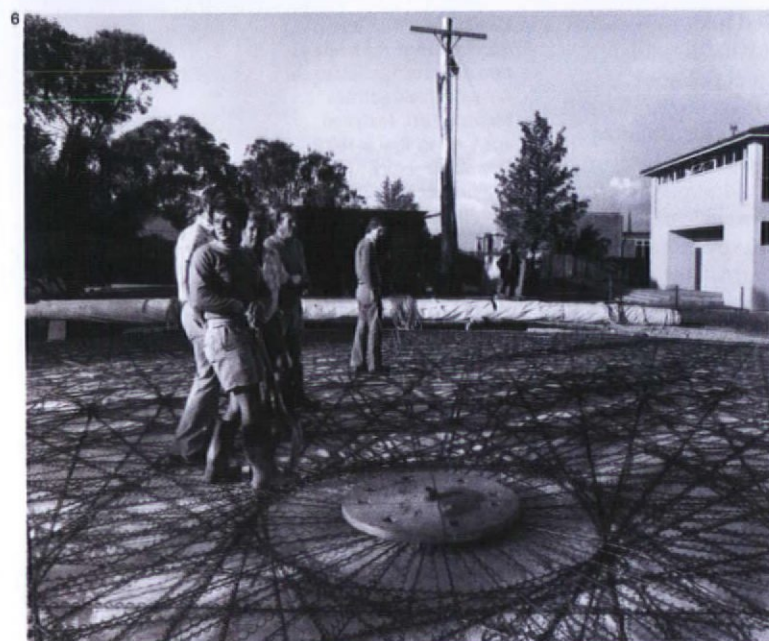
5. A unique system of springs traverse the circular slab, with reinforcement rods inside the springs. The reinforcement is laid over a carefully pleated 'pattern cut' membrane 6. At the centre of the reinforcement mesh a plate is installed from which the concrete vibrators/compactors will be attached
