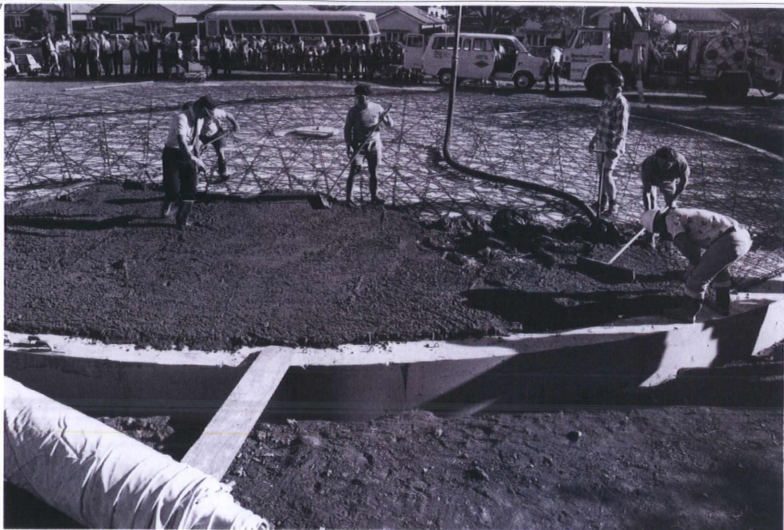
7. Concrete is distributed flat over the inflatable membrane and reinforcement 8. Slump-testing concrete samples on site by Dante Bini (wearing hat)
