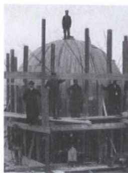
Above: the pioneering (and illegal) reinforced-concrete structure of Saint-Jean-de-Montmartre, Paris (Anatole de Baudot, 1894-1904), was highly controversial
