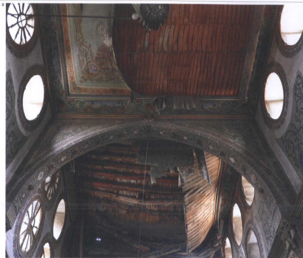
7. Interior elevations and ceiling plan of the public reception room 8. Detail of the faded decorative panelling 9. The deterioration of the roof is causing the ceilings to slump and crack into the room below, revealing the layers of construction and exposing the fragile interior ornamentation to the elements 10. Poplar beams are finely painted in muted greens and pinks
