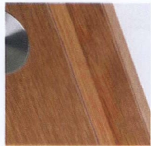
Doors are rebated at the edges to give a flush external surface.
