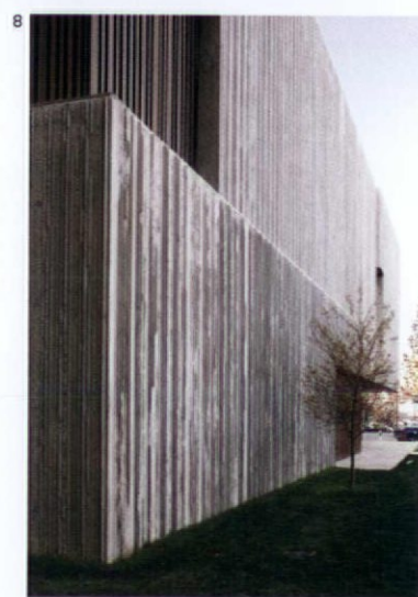
7. Early massing model showing the building's relationship to site, as well as a sense of the ribbed and riven external walls 8. Detail of facade. Concrete was allowed to leach out of the formwork to create the roughly bevelled texture
