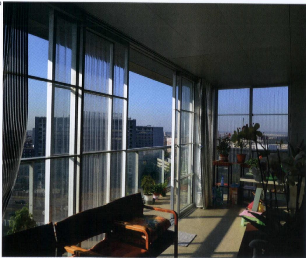
9. A typical dingy apartment interior before the refurbishment 10. New winter gardens and balconies open up the flats to light and views 11. The original poky fenestration is replaced by floor-to-ceiling glazing. Winter gardens can be colonised as tenants choose and the 2m wide space also forms an environmental and acoustic buffer zone
