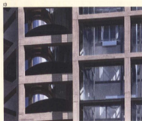
12 & 13. New spiral escape stair clad in stainless steel and playing with the frame 14. Instead of repeating the brick infill, solid parts have been clad in coloured anodised aluminium panels to give the concrete building a new image
