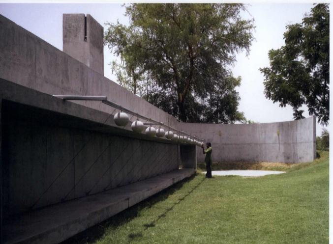
Previous page\_ Metal shutters operated by a system of spherical counterweights open up the garden facade. A roof terrace provides a vantage point Above left\_Concrete wall planes frame the entrance Above\_Detail of the concrete counterweights. The metal shutters are appropriated from agricultural buildings Left\_Shutters in closed mode. As the house tends to be used just at weekends, it needs to be easily secured
