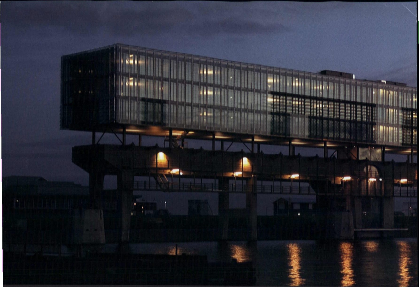
Kraanspoor Amsterdam - 6.000 m 2 glastec louvers - double skin facade - GREEN BUILDING AWARD at the MIPIM 2008
