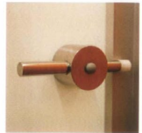
Oasis lock on reverse of Paris CDG's outward opening doors.
