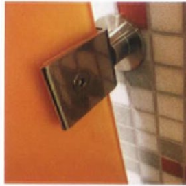
Redesigned bracket to ensure desired gap between wall and glass dividing panel.
