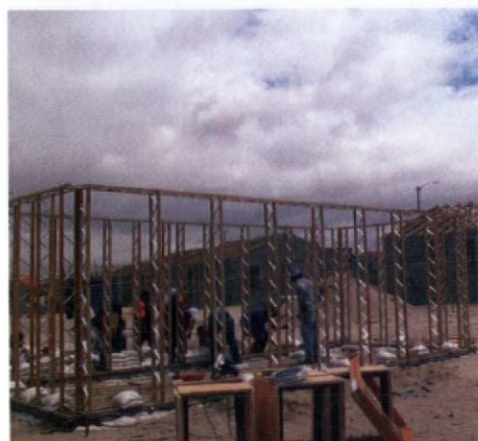
Erecting the frame.
