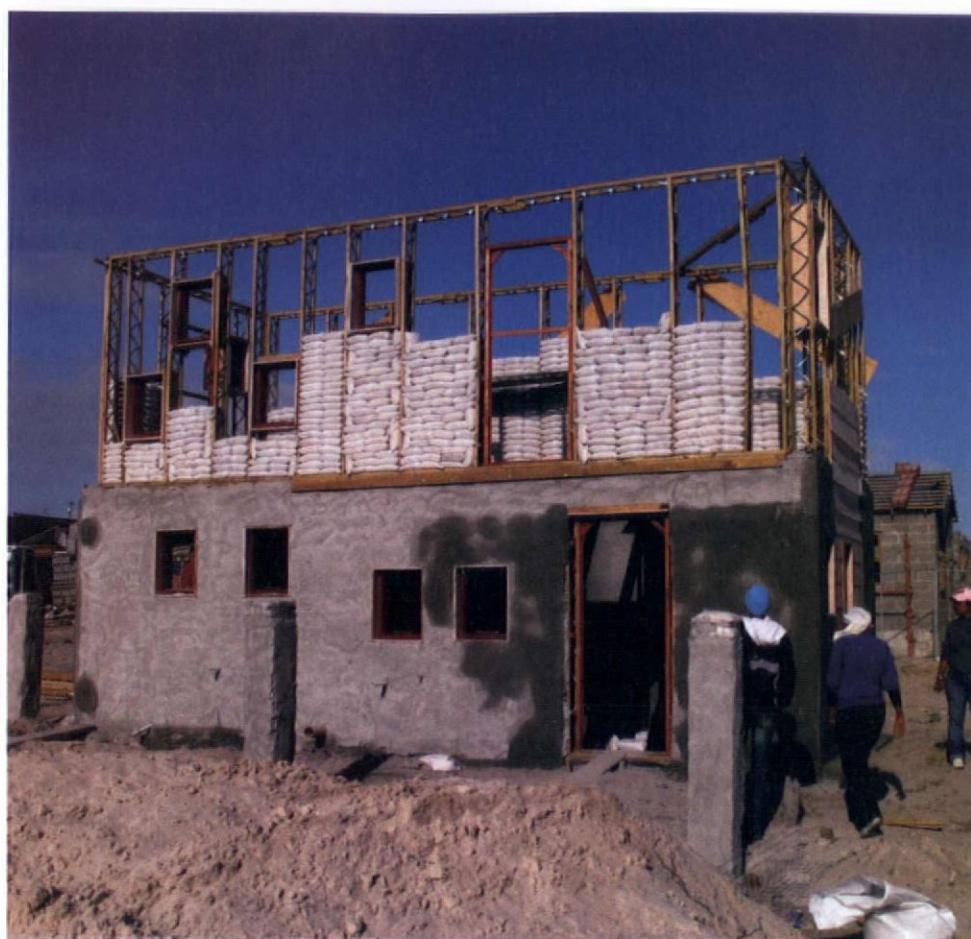
Constructing the upper storey.
