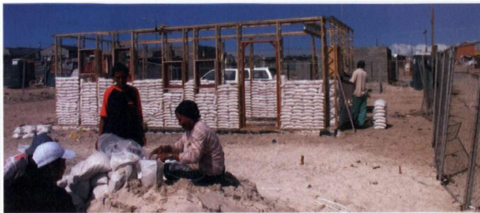
Filling sandbags and stacking them into the wall.
