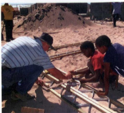
Setting out the frame.
