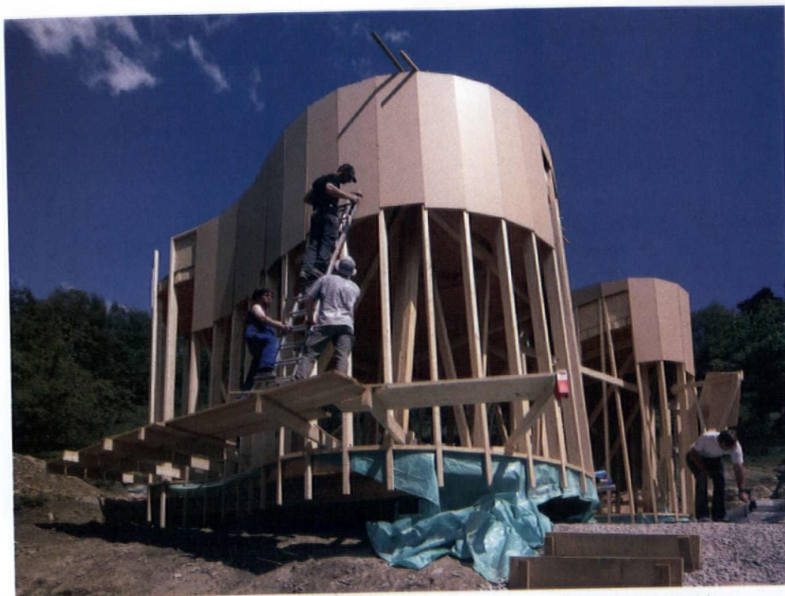
Constructing the external walls. The studwork frame changes angles to cope with the floor and roof plate geometries.
