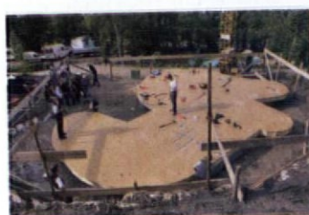
Assembling the flat plate floor.
