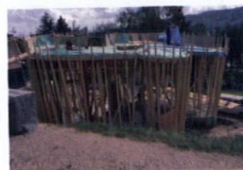
External wall studwork in progress.
