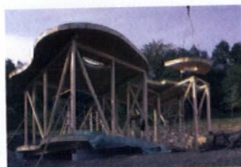
Roof plate in position.
