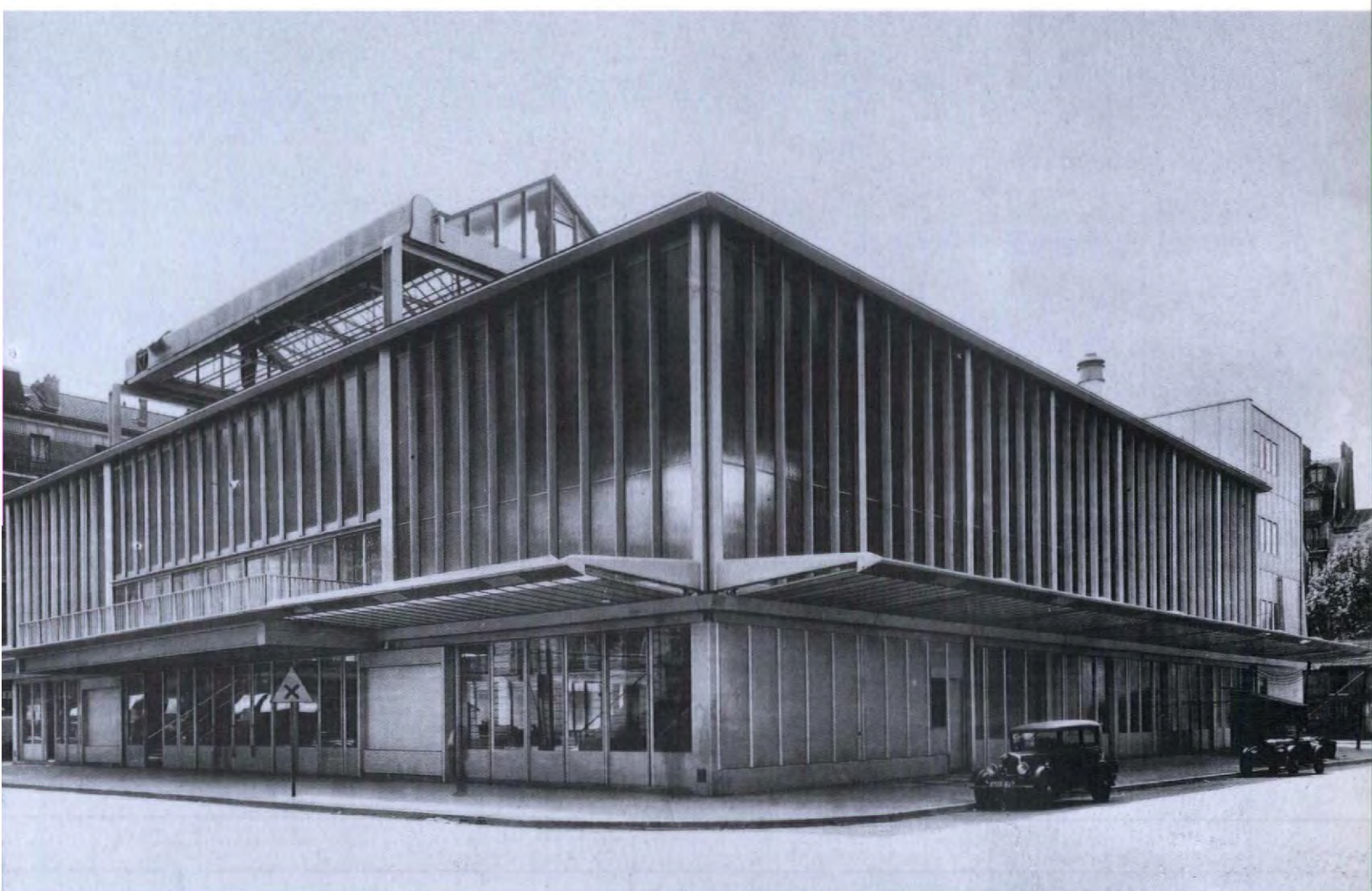
Maison du Peuple in the Paris suburb of Clichy, 1936-39. Designed with architects Beaudouin & Lods, it had stressed-skin wall panels and huge internal moving parts.
