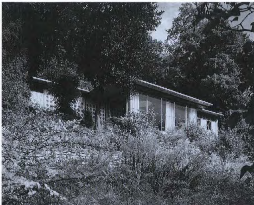
Prouvé's house built on the hills overlooking Nancy in 1954. No component was heavier than could be carried in a Jeep. House open to the public until mid-October. (Photographs above and bottom right are by Martin Charles.)
