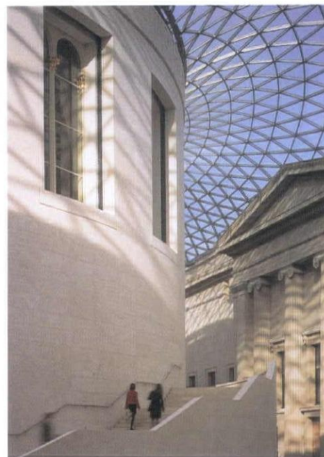
Sydney Smirke's rotunda was never intended to be seen from the outside and has been refaced in stone.
