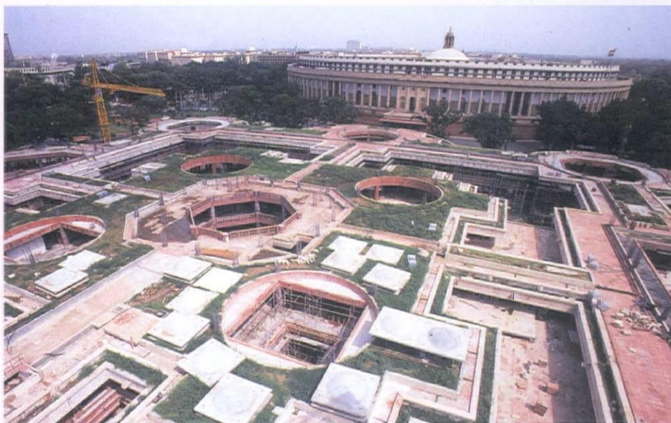
Raj Rewal's Parliament Library adds to the great Lutyens/Baker complex. Under construction and ...
