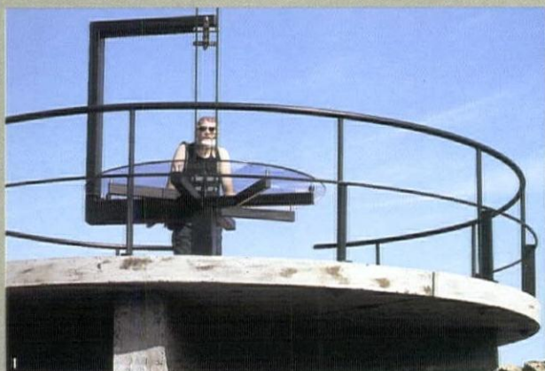
ar+d HIGHLY COMMENDED VIEWING PLATFORM, SOGNEFJELL, NORWAY ARCHITECT CARL-VIGGO HØLMEBAKK
