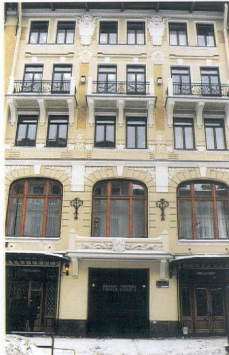
The former Civil Engineers building from 1904 at Serpuhovskaya street, bordering the St Petersburg city centre, was a ruin when a small developer decided to put time, money and energy at stake to renovate the house with an outcome that pleases everybody.
