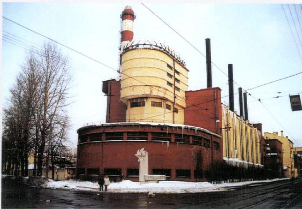
St Petersburg architectural heritage includes this textile factory at Pionerskaya street, on the Petrograd side, which still conveys a dynamic, pioneer design by Erich Mendelsohn in 1927.
