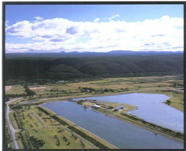
REGATTA CENTRE, SYDNEY, AUSTRALIA ARCHITECT WOODS BAGOT
