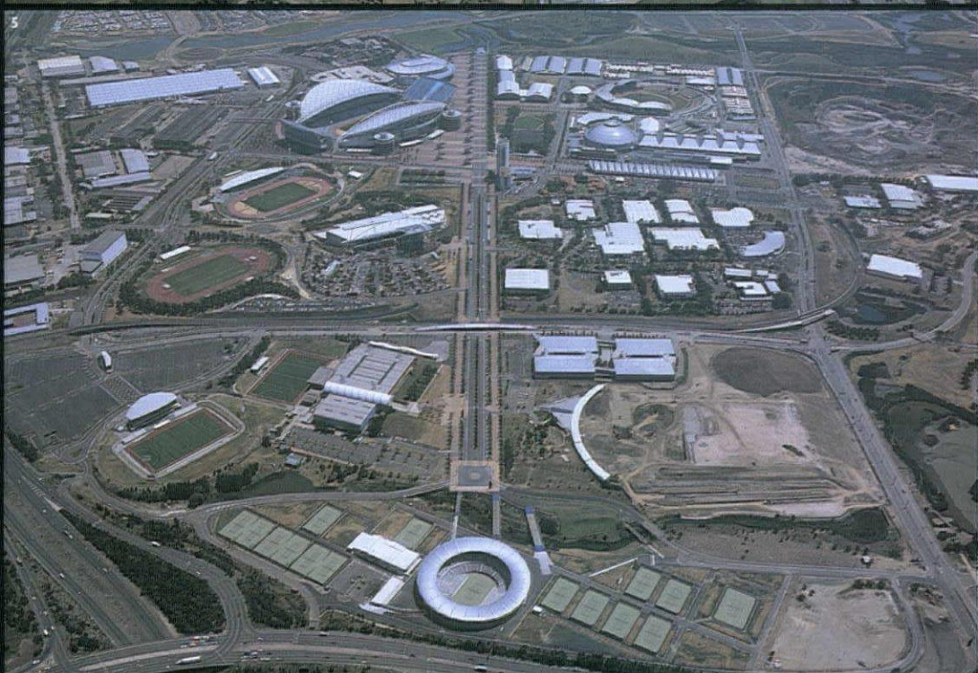
4 Looking down Nield's cardo from north with Sydney Superdome (p57) and Stadium Australia (p54) right. 5 Looking north up the cardo, with tennis centre (p60) in foreground.
