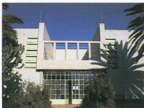
Formerly the first hotel in Asmara, now public offices. Clean geometry and white walls have a nautical spirit.
