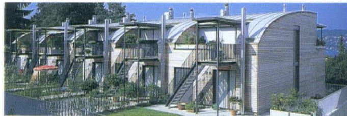
Object residence "Seepark Wannen"
