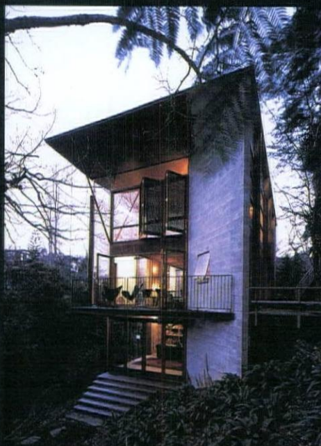
1 From north, with 45 degree concrete block blade.
