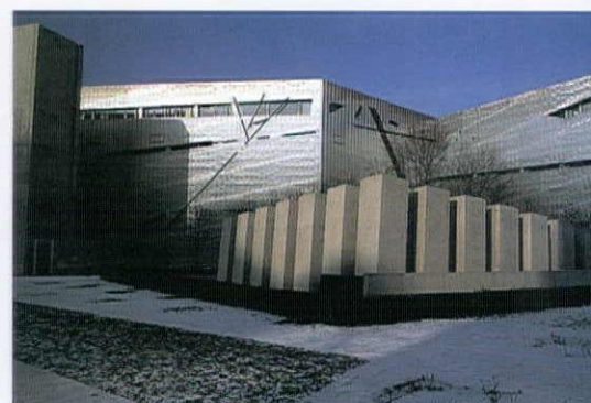
Libeskind's leaning columns at the Jewish Museum.
