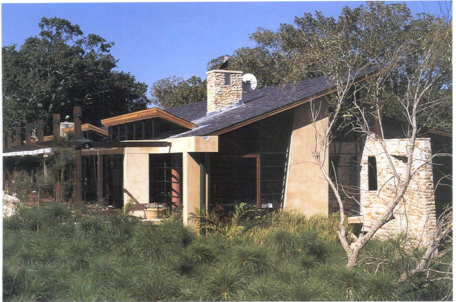
VISITORS' CENTRE, CAPE TOWN, SOUTH AFRICA ARCHITECTS GAPP ARCHITECTS AND DAVID B. LEWIS
