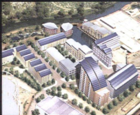
The Peabody Trust had European funding to install photovoltaic panels in a £70m mixed-use development on a 10 acre former gasworks site, West London.
