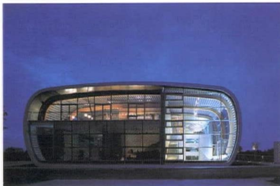
Offices and workshops, Rellingen, Germany (p52)
