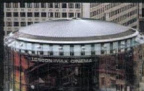
Imax Cinema - London Architect: Avery Associates
