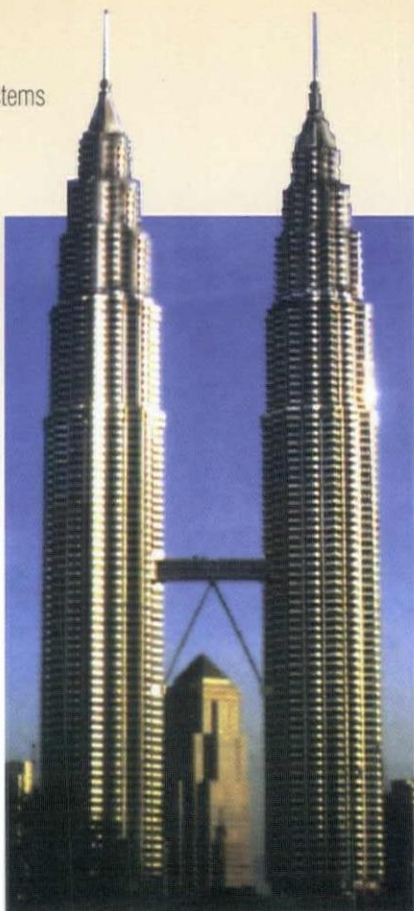
FOAMGLAS® insulation was installed on the chilled water system of the Kuala Lumpur City Centre.
