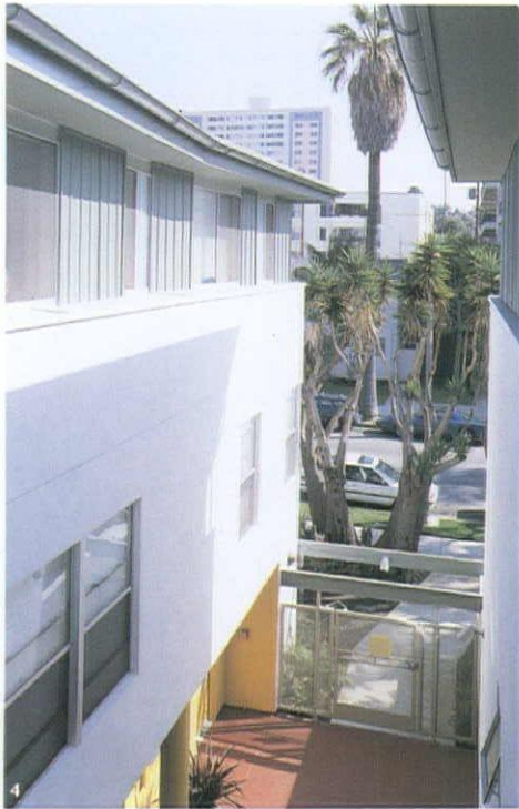
4 A narrow semi-private street leads to the central courtyard. Although public and private realms are separated by a gate, the scheme is not obsessively hermetic in its relationship with the wider world. 5 Kitchens overlook the courtyard, fostering a sense of informal communal supervision.
