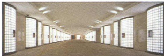
Construction of Chiba Station East Entrance Underpass, Chiba Pattern: Opaline Plain Architect: Chiba City Photo by Hitoshi Kawamoto
