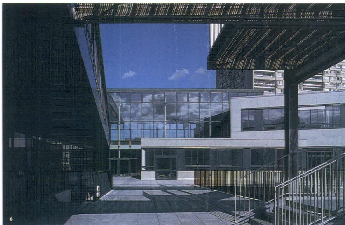
6 Northern end of the site with glass atrium and north end of apprentice centre.
