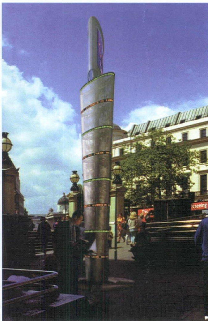
Attractor with elliptical collars clamped on central structural mast.
