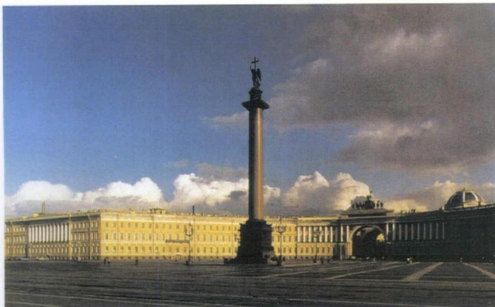
East wing of Rossi's General Staff Building, St Petersburg.
