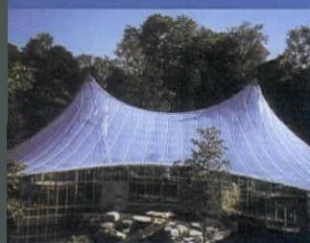
PROJECT: Lion House - Zoo Enclosure MATERIAL: Double layer Velaglas® AREA: 2000 sq/m
