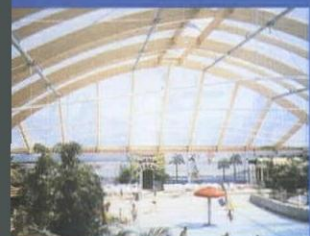
PROJECT: Swimming Pool and Leisure Building MATERIAL: Triple layer Velaglas® AREA: 2200 sq/m
