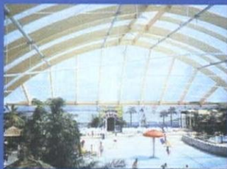
PROJECT: Swimming Pool and Leisure Building MATERIAL: Triple layer Velaglas® AREA: 2200 sq/m
