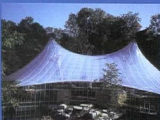
PROJECT: Lion House - Zoo Enclosure MATERIAL: Double layer Velaglas® AREA: 2000 sq/m
