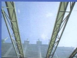
PROJECT: World Economic Summit Building MATERIAL: Double layer Velaglas® AREA: 5000 sq/m
