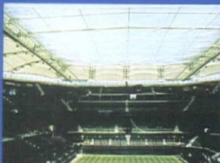
PROJECT: Retractable Tennis Stadium Roof MATERIAL: Double layer Velaglas® AREA: 1400 sq/m
