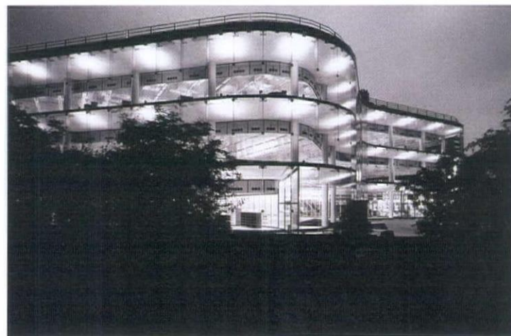
Foster's iconic Willis Corroon building
