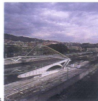
5 Sleekly aerodynamic precast concrete platforms (containing ramps and stairs) provide lateral support.
