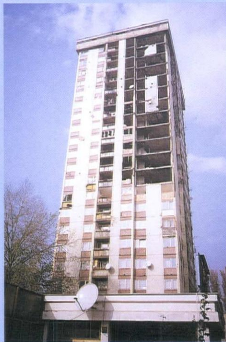
Housing, Zmaja od Bosne: collapse in Sniper Alley.
