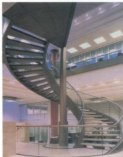
Staircase in glass blasted stainless steel, and curved glass
