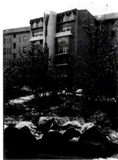
4, 5, canal and court sides of gatehouse building.
