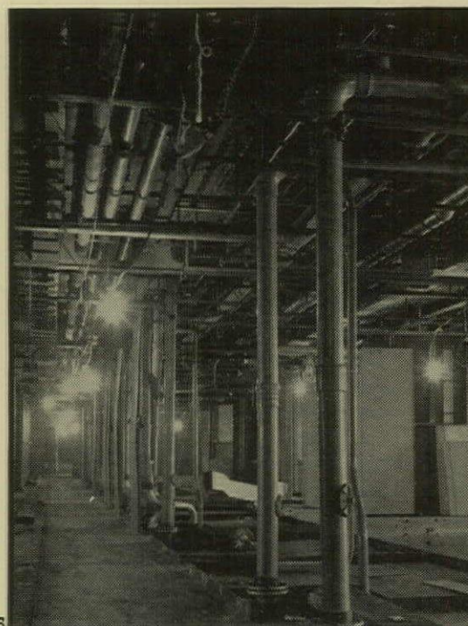
5, services in one of the corridors being built in the passenger accommodation. Perforated beams and unusually strict planning of pipework give greatly improved headroom. 6, the same corridor after completion.
