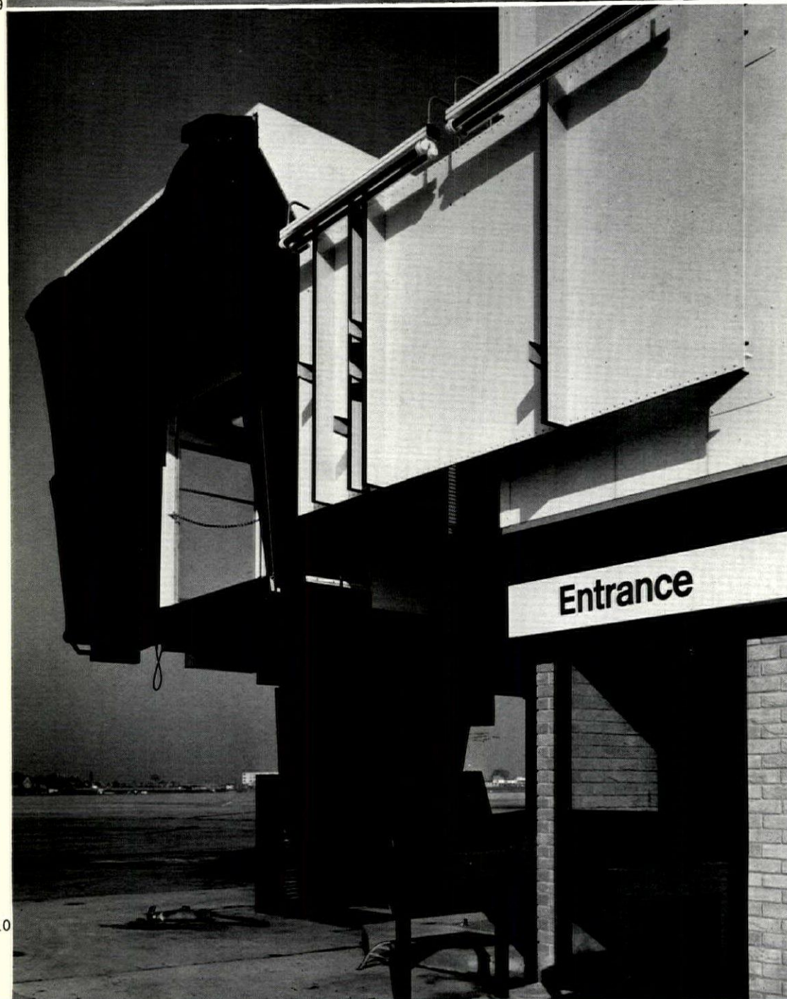
9, air-jetty connecting a forward waiting room (left) with an aircraft. 10, front of an air-jetty, with nose-in guidance board on the right.
