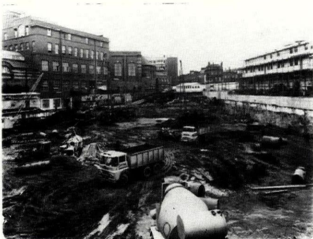
Unstrutted Cantilever Diaphragm Retaining Wall along the perimeter of the excavation for the extension of the City University, London
