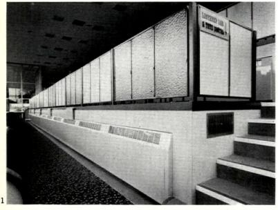
grille formed from extruded sections. Electrical ducting is made for in-stallation below the heating units. This has a sloping top to allow the free entry of air into the heater and is made with either two or three compartments so that mains supplies, telephones and other circuits can be kept separate. Socket outlets can be arranged in the ducting itself or at high level in the heater units. Copperad Ltd., Colnbrook, Bucks.
