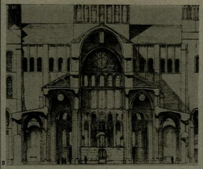
5, cross section of the nave of the third Abbey Church of Cluny as originally constructed without flying buttresses to the main vault. These were added after the vault collapsed in 1125.
