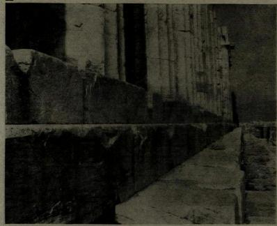
22, the vertical curve of the stylobate of the Parthenon. Other refinements include similar vertical curves in the superstructure, entasis and inclinations of the columns, slight thickening of the corner columns in relation to the others, and other slight inclinations.
