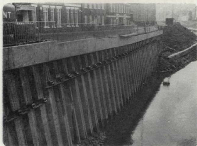
Sheet piling tied back by means of pre-tensioned anchorages at the new Nene Quay, Wisbech
