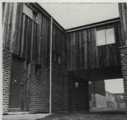
(Below) One of the varieties of cladding employed at Bicester—brick and vertical rough-sawn cedar.
