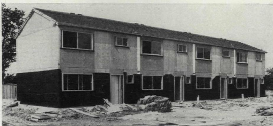
(Above) An early stage of construction at Bicester—framework, plywood skin and roof completed, ready for final cladding and interior finishing.
