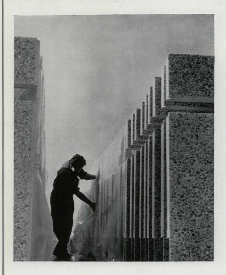
Precast concrete cladding and structural units.
