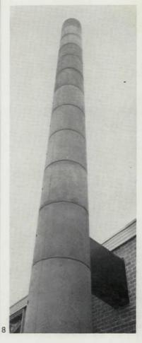
surface. The units are made in standard 4-ft. lifts and are quick to erect. By extending the system combined water tanks and chimneys can be provided in a variety of forms.
