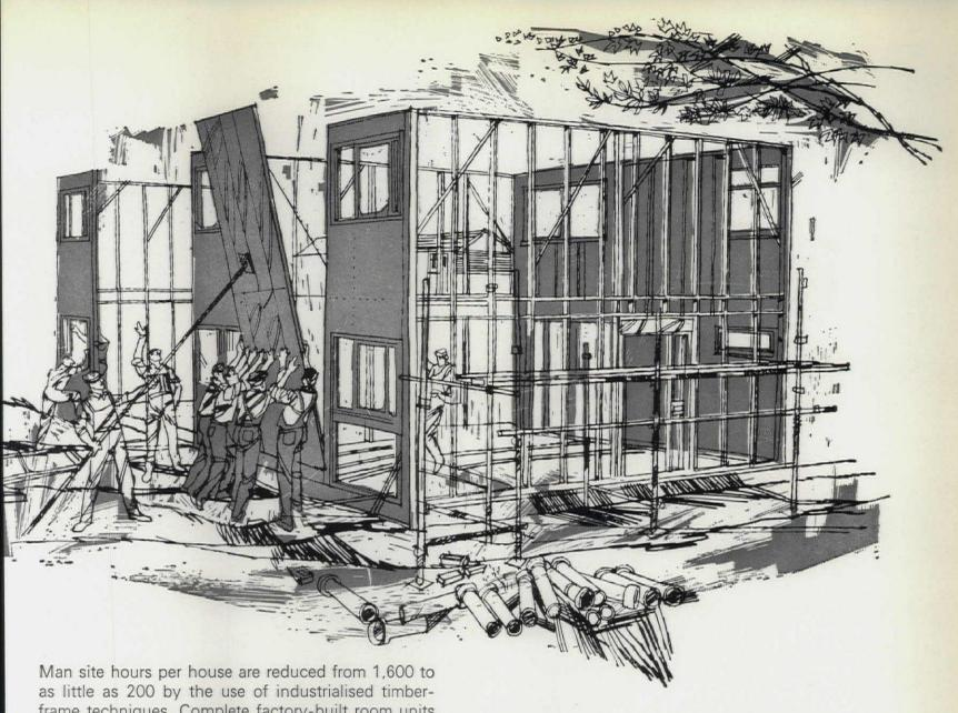
frame techniques. Complete factory-built room units can be assembled, giving an average time of about two days for completion of a house. Or roof, wall, floor and other factory-produced components can be assembled on site with phenomenal speed. Timber-frame methods can be used for housing developments of any size—the smaller builder can adopt a timber-frame system just as easily as a large contractor and so benefit from its tremendous advantages.
