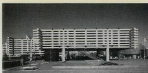
21, Japan: cage of prestressed beams over an open ground floor.
