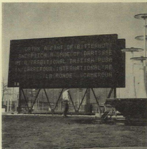
3, information display board: one of several in the exhibition grounds, all electronically controlled from the Operations Control pavilion.
