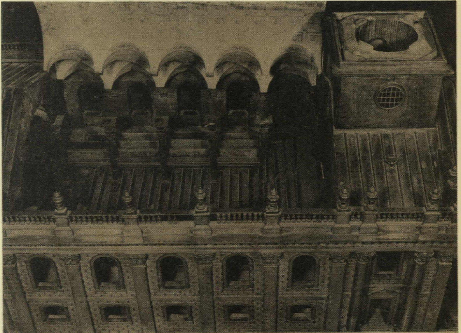
11, this model for St. Martin-in-the-Fields (erected between 1722-6) is the most elaborate example in England next to the Great Model. Made of pine and mahogany to a scale of 1 in. to 4 ft. for £71, it represented every aspect of the design for the consideration of the Commissioners. When the two parts of the roof are removed, 12, the complete features of the interior are revealed, even to the proposed form of plaster decoration for the vault. The right-hand part of the roof can be removed to show one of the four staircases extending from gallery level to the crypt.
