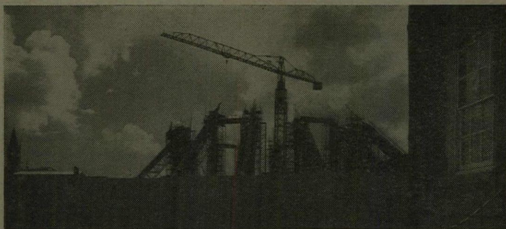
2, the cathedral under construction in 1963, showing the centrally-placed tower crane. The contractors were brought in at an early stage; the buttresses and the ribs of the cone were redesigned to an equal length so that the same formwork could be used for both.
