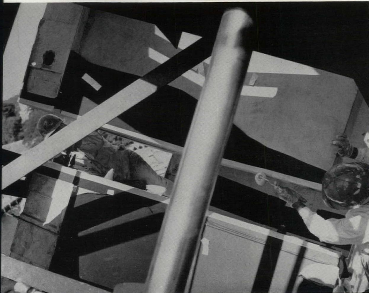
1, Sydney Opera House, 1965 (J. Utzon, architect; Ove Arup and Partners, consulting engineers). Preparation of the joint of a precast concrete element for bonding with epoxy resins.
