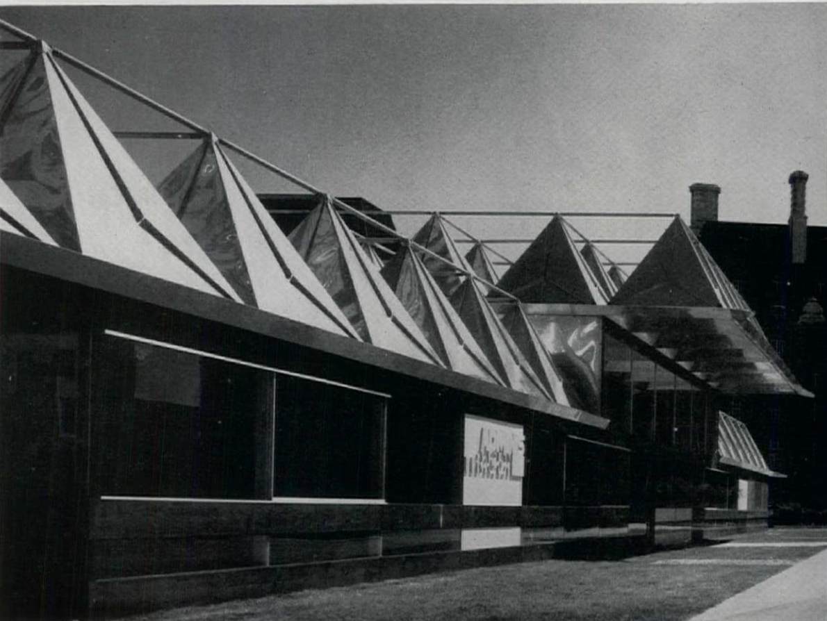
9, footbridge with chords of laminated timber construction. Muirhead & Sons Ltd. 10, IUA Congress building, London 1953 (architect, Theo Crosby; engineer, Professor Z. Makowski). An extremely light roof structure of 108 aluminium pyramids bonded with epoxy resin and fabricated by British Aluminium Ltd. and Marshall Motor Bodies Ltd.
