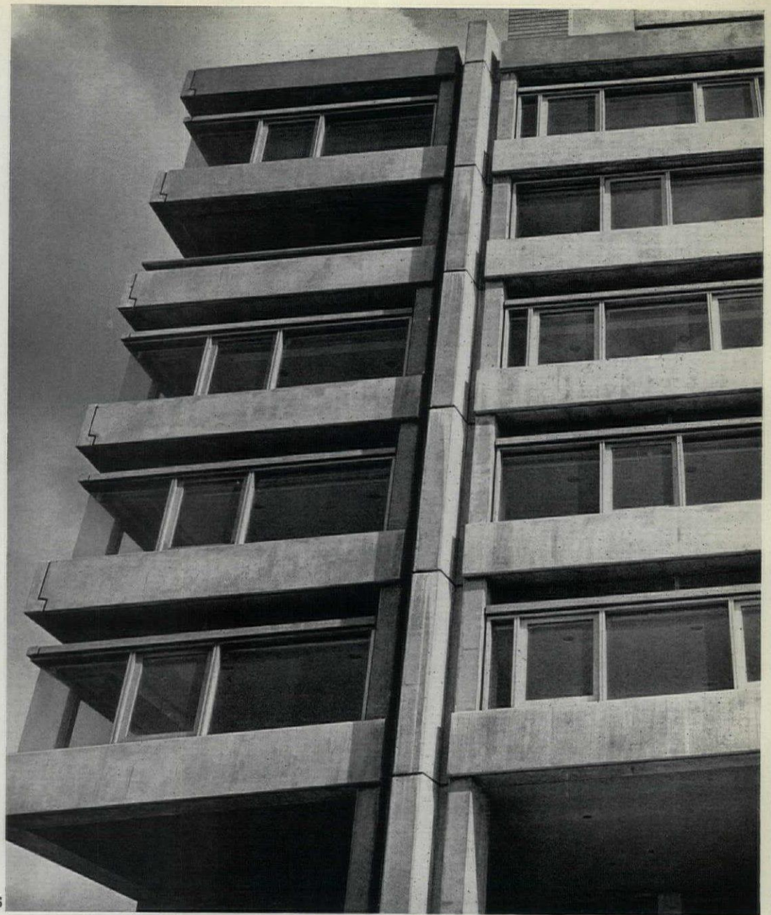
5, precast duct and spandrels on the first to fifth floors.
