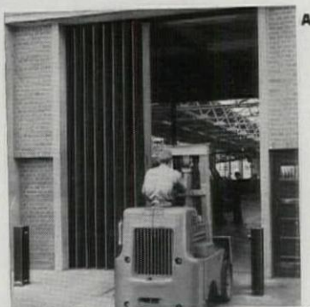
A A factory installation of Bolton photo-cell controlled Shutter Doors.
