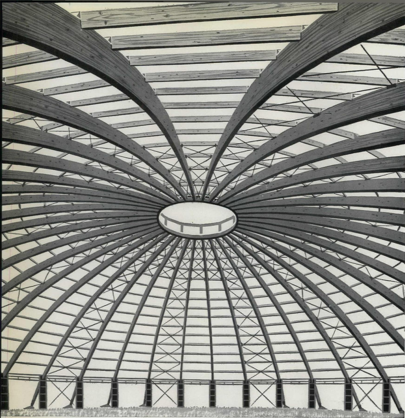
Laminated timber beams in 206-ft diameter sports hall at Newcastle-upon-Tyne Lightfoot Centre. Architects: Williamson, Faulkner Brown & Partners. Structural Engineers: Cooper, Higgins & Partners.
