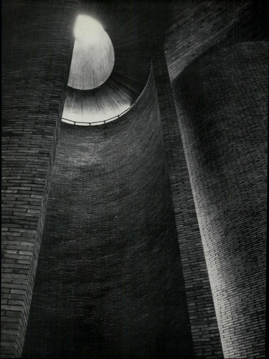
Plain cylinders of brick form the whole wall structure of a recently completed church at Todi, near Perugia, by Julio Lafuente. As the plan shows, each cylinder contains a chapel, opening to the nave. The photograph opposite looks upward to the rooflight that crowns each chapel—more illustrations on pages 221-223.
