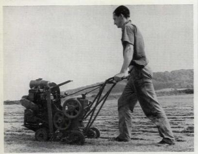
2, the Ryan Turf Lifter can cut turves ten times faster than the most skilled hand.
