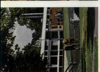
National Service The Nenk method of industrialised building rationalises the construction process for a wide Rapidly erected steel-frame structures have space-frame' roof and floor decks formed of buildings for the Services. from easily handled and erected steel pyramidal units. Steel is also used for columns. and in staircases at Maidstone Barracks. Steel on range
