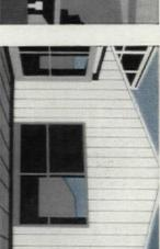
tive plastic-coated steel sheet cladding panels give a pleasant 'boarded' effect on struction times and costs. and because it is speedily fixed cuts con-Formed from pre-finished steel sheet, panel-Maintenance-saving colour finish Attracthis new Hereford County Secondary School.
