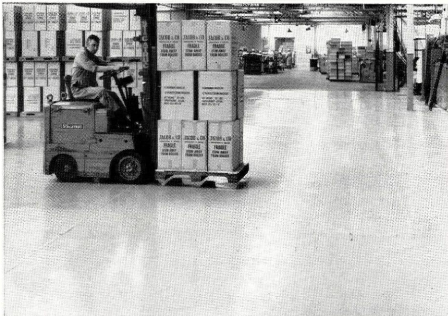
ABOVE. This high-gloss, non-slip hygienic floor was laid by Protective Materials Ltd. of Birmingham at the Aintree factory of a leading biscuit manufacturer, using Bibby Merginamide in the epoxy-resin hardener.
