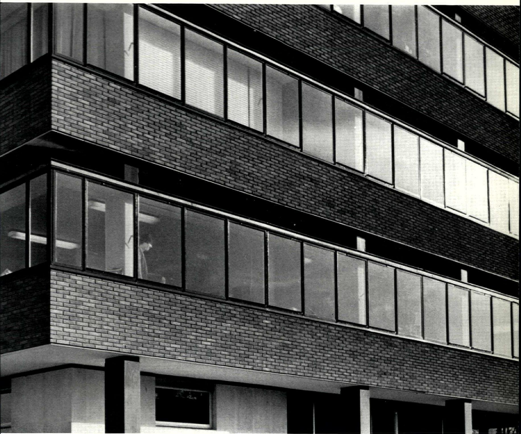
1. detail of south elevation, showing the expression of each office floor as a continuous glazed box, threaded through by the perimeter columns.
