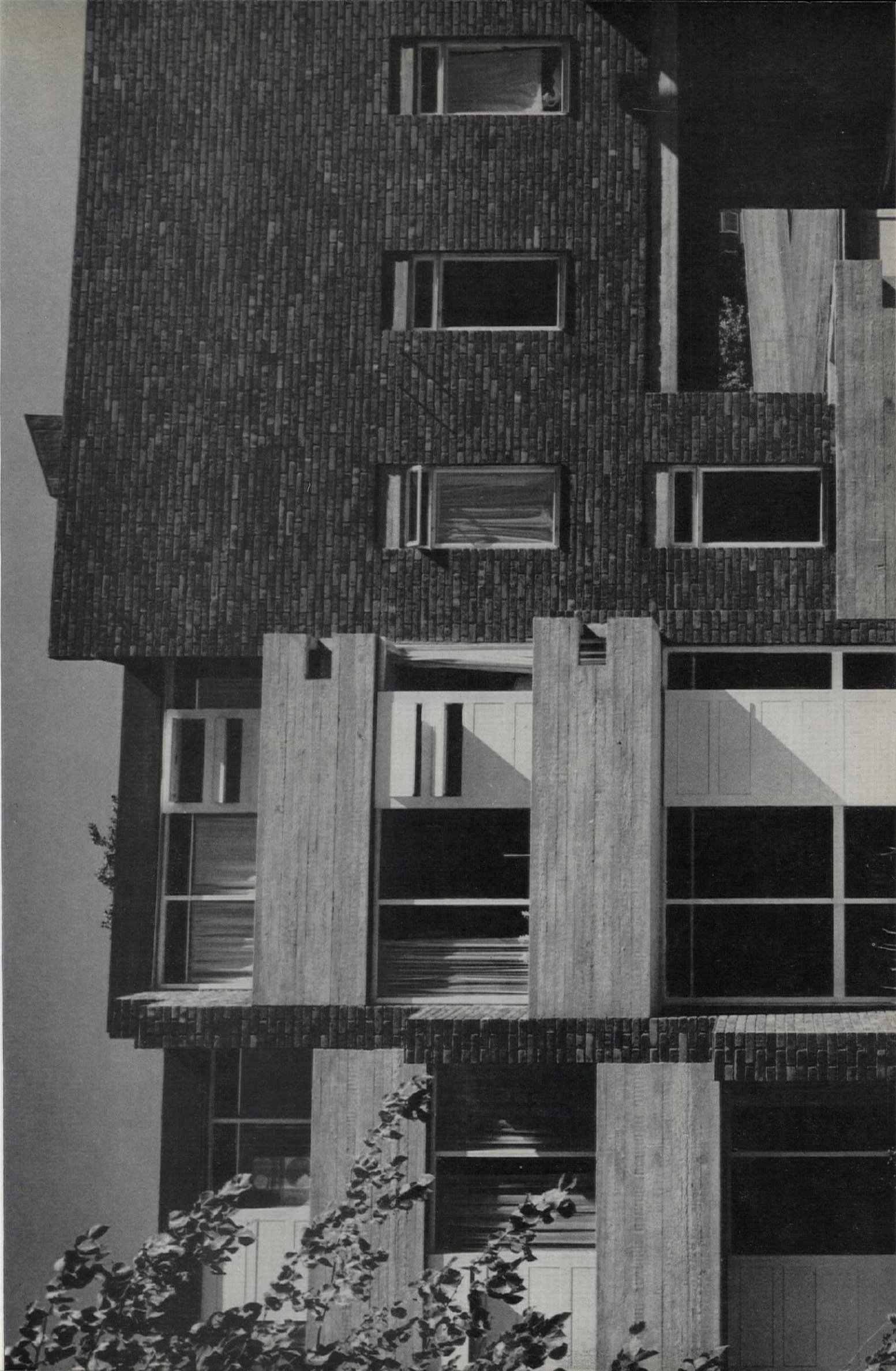
5, detail of elevation of north-west wing, showing texture of boarded concrete and facing bricks with raked joints. Main entrance ramp is seen through arch.
