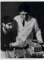
5, St. Anne's Redevelopment, Rotherham. To provide consistent detail finishes as would obtain actual buildings, the complete elevational pattern of ribbed concrete surfaces, glazing and colour detail was reduced to mode scale and mas produced from a master, then applied to building cores. (Architects, Gillinson, Barnett & Partners.)
