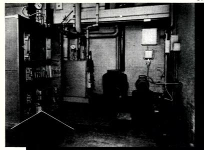
Automatic movement of fuel from bunker to boiler leaving floor space unobstructed
