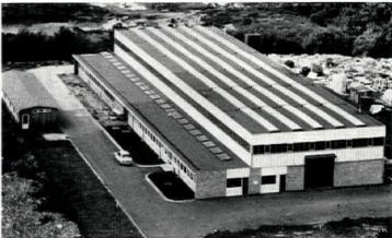
The Tri-Light roof system is a package deal "Umbrella". Our quotation includes the complete steel frame, the roof decking, diffused double glazing units and the asbestolux board covering all internal steelwork.
