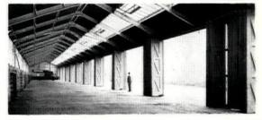
'TANGENT' Top hung and bottom roller gears for doors sliding round corners and folding
