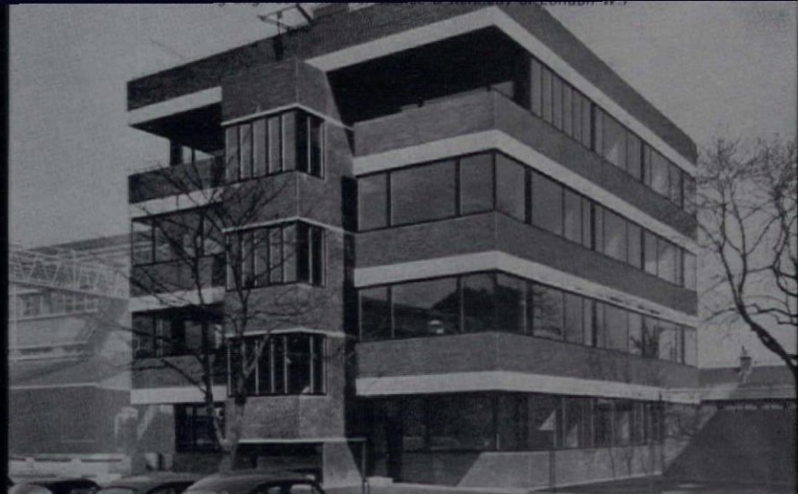
ALUH windows in this building incorporate sealed double glazed units. Most are fixed lights but some side hung sashes are included. The aluminium facings are etched and anodised BLACK and the timber frames are of Douglas Fir.
