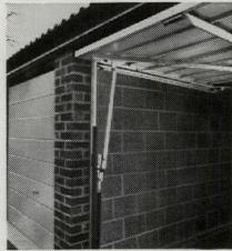
THE CARDALE garage door is delivered on site as one unit, which can be installed in 15 minutes. The metal frame can be fixed directly to brick or metal or to the normal wooden door-posts. And the Cardale door has a strength-to-weight ratio previously thought impossible! (Slide-away door by Cardale Doors Limited: Dragonzin galvanised steel by The Steel Company of Wales.)
