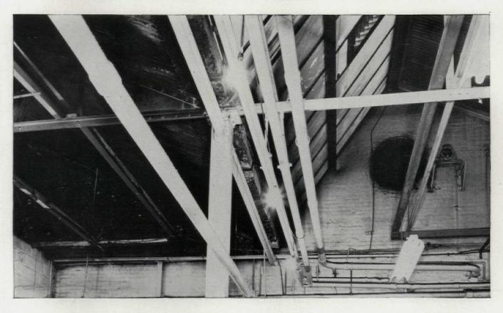
The smoke staining of the roof and gable walls, clearly visible in the photograph taken at the Acton Works of Wilkinson Sword Ltd. the morning after the fire, shows how Colt Fire Vents work.
