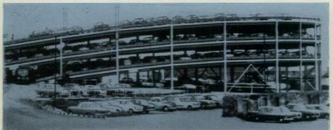
Quick solutions—in steel Many multi-storey steel car parks are easily dismantled and reerected, and can thus meet temporary demands for central area parking on vacant sites during
