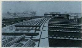
Steel elevated road Fylde Junction Higher Bridge at the 3-level Broughton M6—A6 traffic interchange. This attractively designed welded steel box girder viaduct, supported on steel piers, has a curved length of 1,300 ft. *The Structural Deck* (above) comprises a 14 ft. wide, 8 ft. deep, three-cell welded spine beam with 14 ft. long cantilevers on each side.
